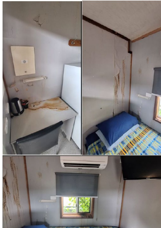
VAC 2 Room – Result of condensation buildup. No windows left open.
