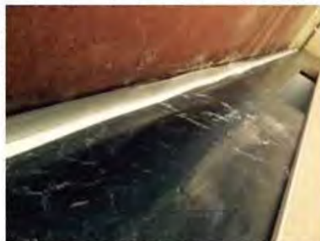
A bead of "Sikaflex" is applied to join of the stainless-steel plate and the bench top, then the splashback is put in position
