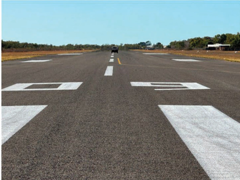
Photograph 1. Typically sound runway pavement.
