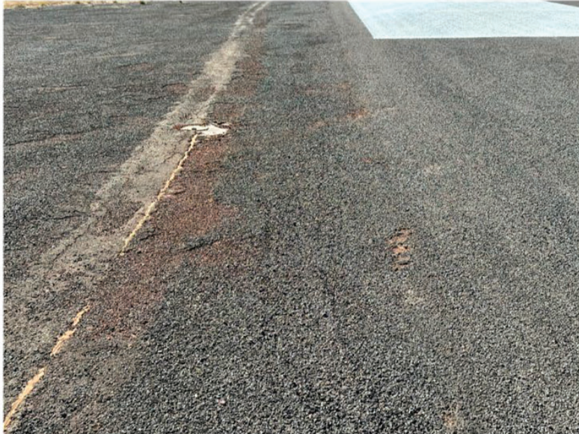
Photograph 4. Example of edge break aways at the intersection with the old cross runway.
