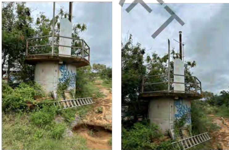
Figure 16: SPS C Compound
