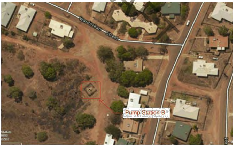
Figure 2: Pump Station B
