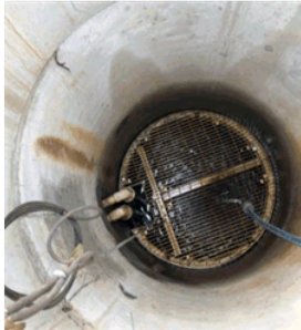
Dauan Wells Upgrade Dauan Island, Queensland
