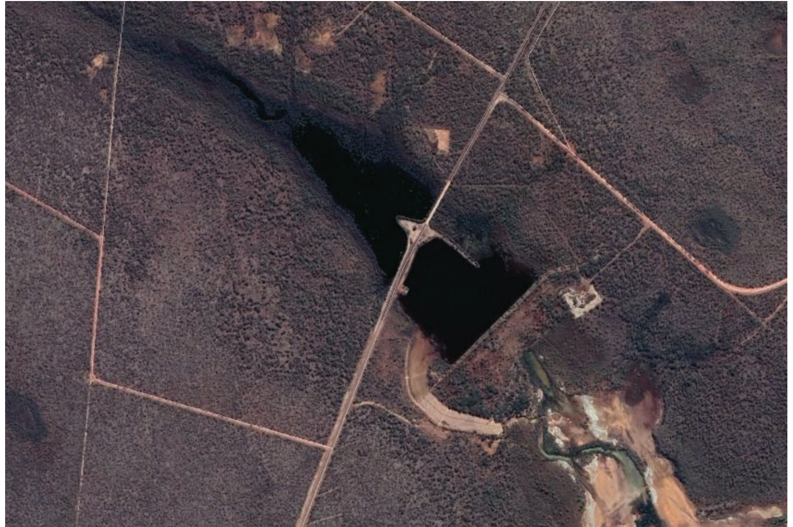
Figure 7: Dithery Creek Dam (Source: Queensland Globe)
