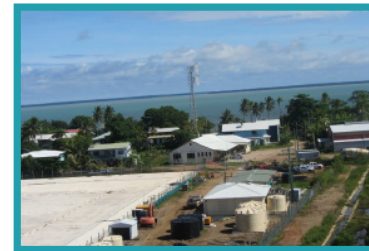
Industrial sheds and laydown area
