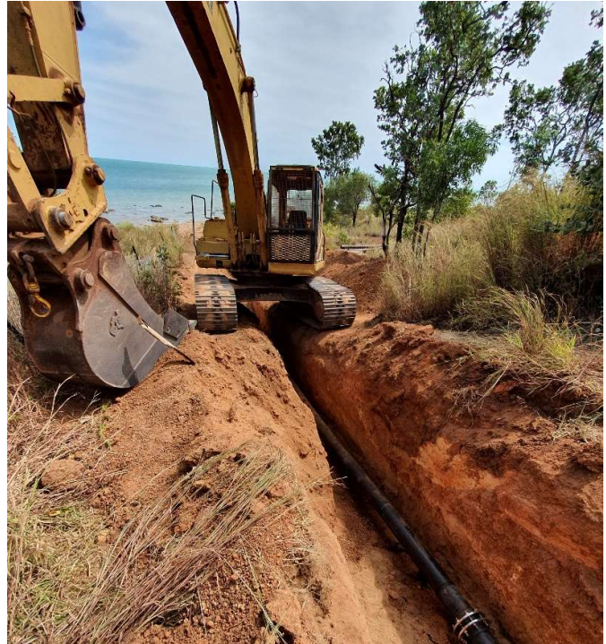
The above photograph is during construction of the new outfall pipe.
