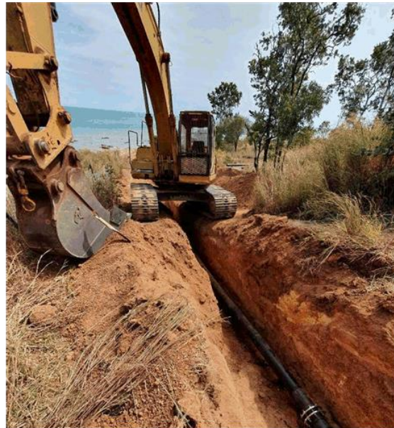
The above photograph is during construction of the new outfall pipe.
